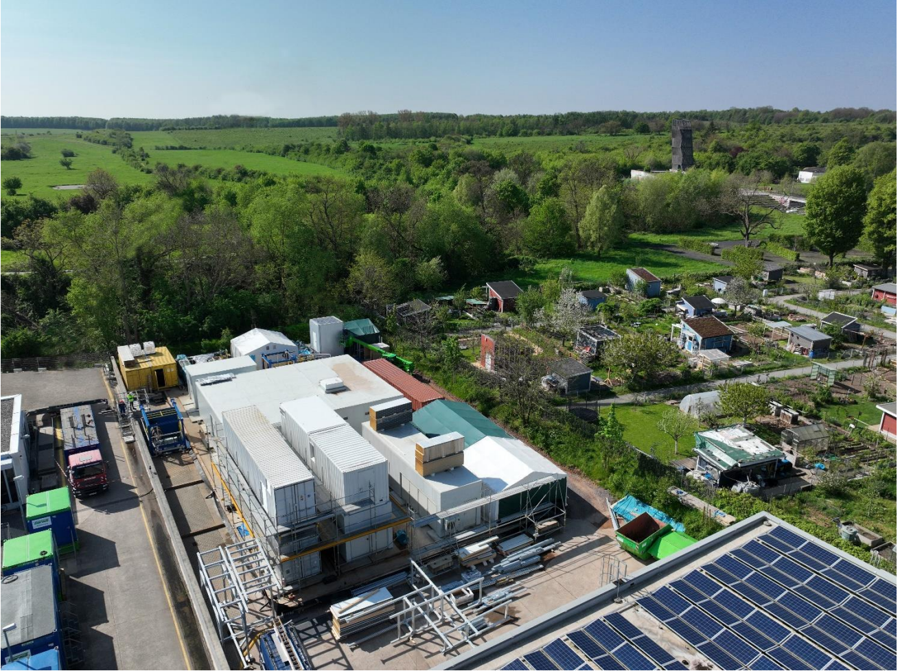
Figure 1. Vulcan's Lithium Extraction Optimisation Plant at Landau
